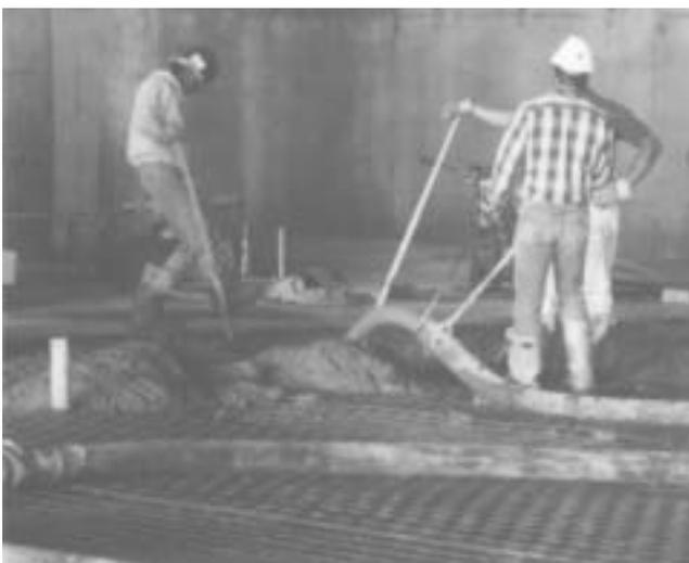
*Workers ensure the proper WWR cover as they work with the pumped concrete.*
