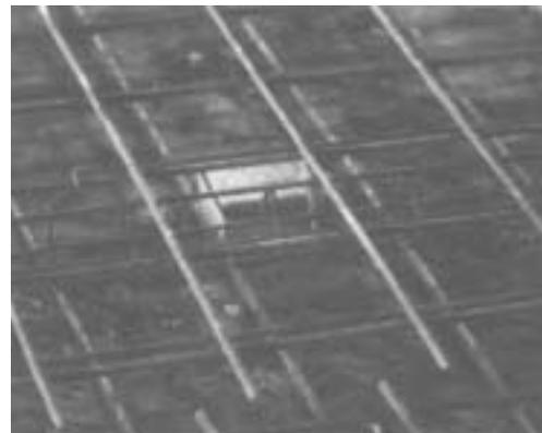
*Here concrete blocks support the bottom layer of WWR and continuous wire chairs support the top layer.*
