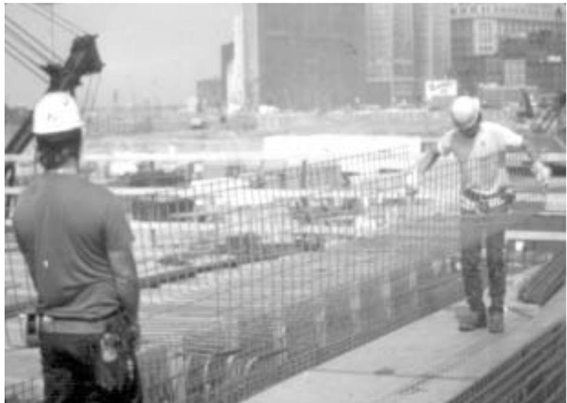
*Bent cages of WWR for shear reinforcement in the poured, in-place concrete girders are easily handled by two workers.*
