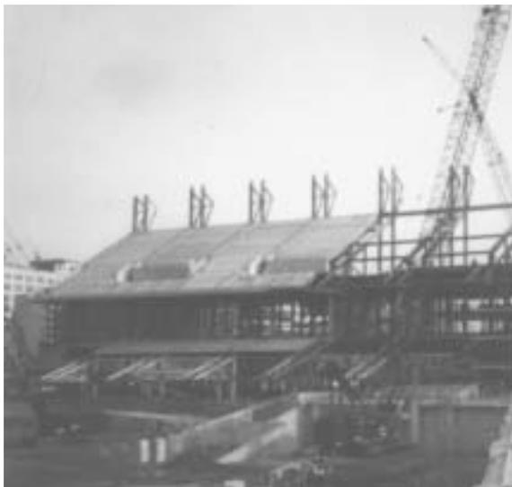
*Precast concrete tiers for seating are reinforced with sheets of welded wire reinforcing.*
