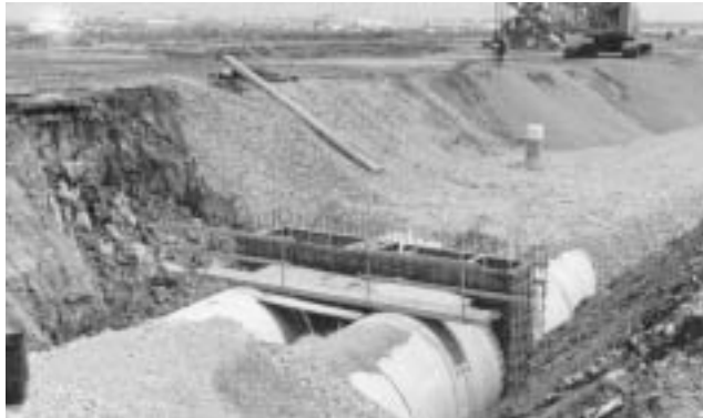
Inlet structures were formed with steel reinforced concrete.
