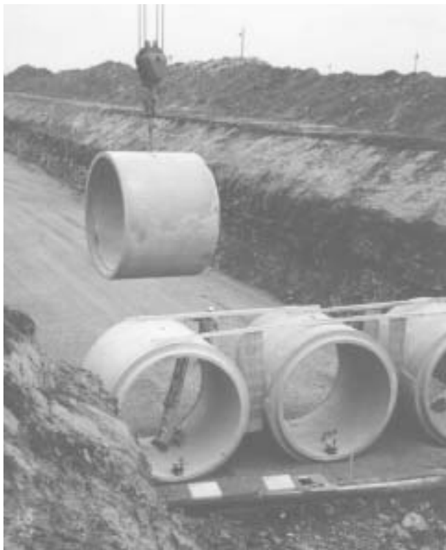
Well prepared grade and proper alignment is essential before installing pipe.
