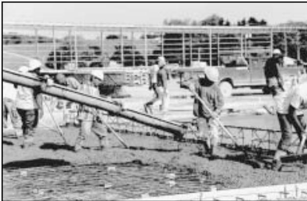
*Workers walk on or into wide spaced welded wire reinforcement without deflecting or displacing it during concrete placement.*
