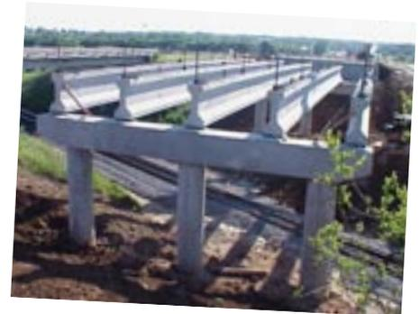
of State Department of Transportation (DOT) projects now choose welded wire reinforcement for bridge girders. WWR, along with pre-stressed steel strands, are now frequently used in standard beams and girders.
