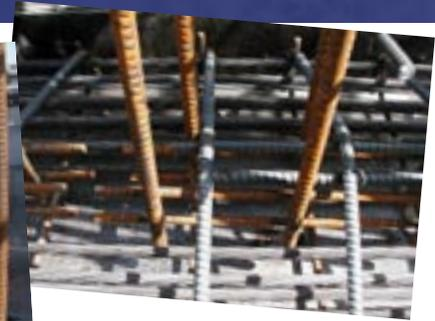
Idaho DOT works on 87 bridge girders using welded wire reinforcement.
