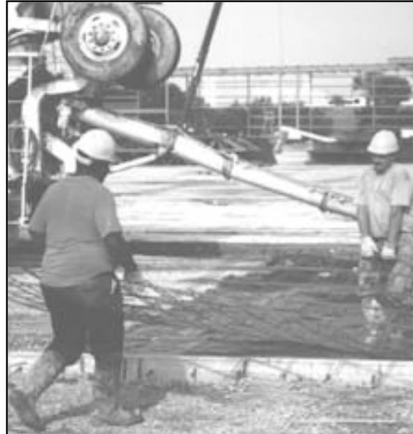
*"With welded wire you don't have to prepare it — it is already welded together — you pick it up and set it in place and continue the pour"*
