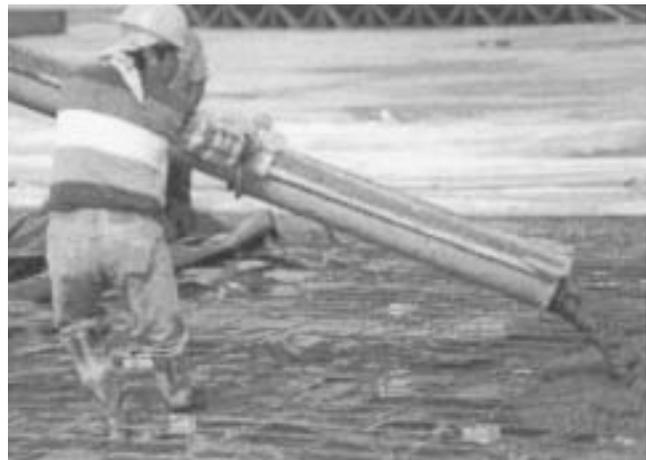
Workers walk on or into wide spaced welded wire reinforcement without deflecting or displacing it during concrete placement.
